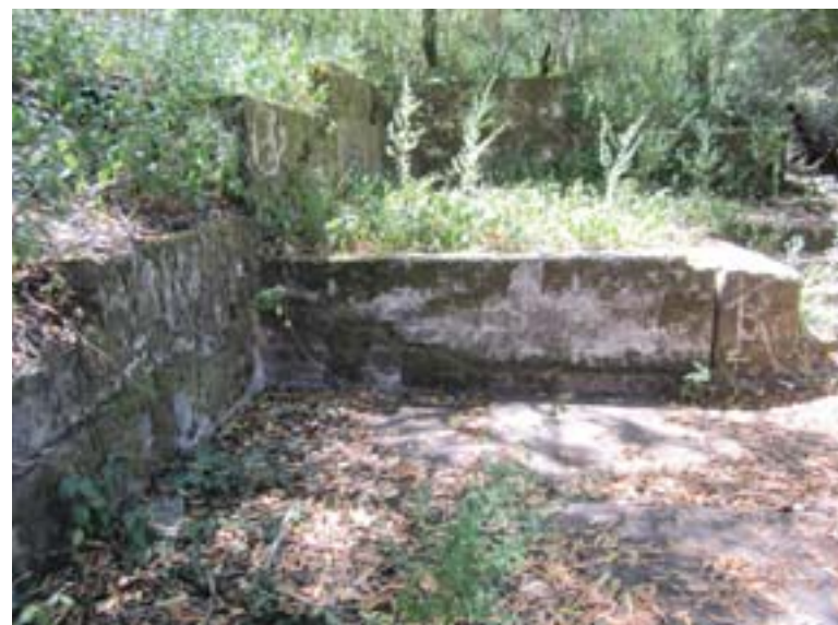
A home's foundation
